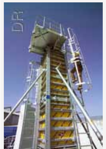
Fig. 1 Coffrage poteau DOKA
